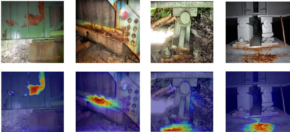
Fig. 25. Robust detection under low-light and reflective conditions. Left: preprocessed input; Right: activation map (warm = high response).
