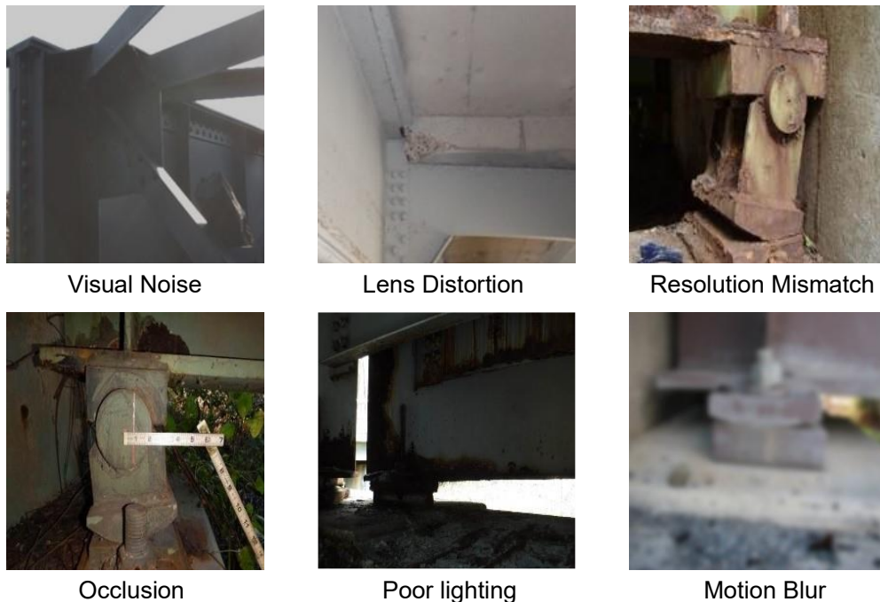
Fig. 4. Sample images illustrating common quality issues such as glare, occlusion, rust artifacts, vegetation obstruction, poor lighting, and motion blur.
