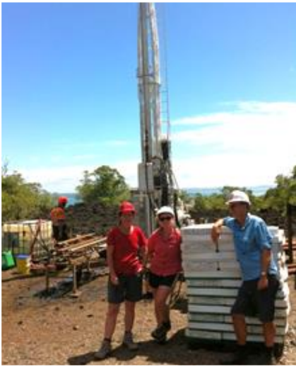
Figure 21. Drill site on Rangitoto Island, February 2014.
