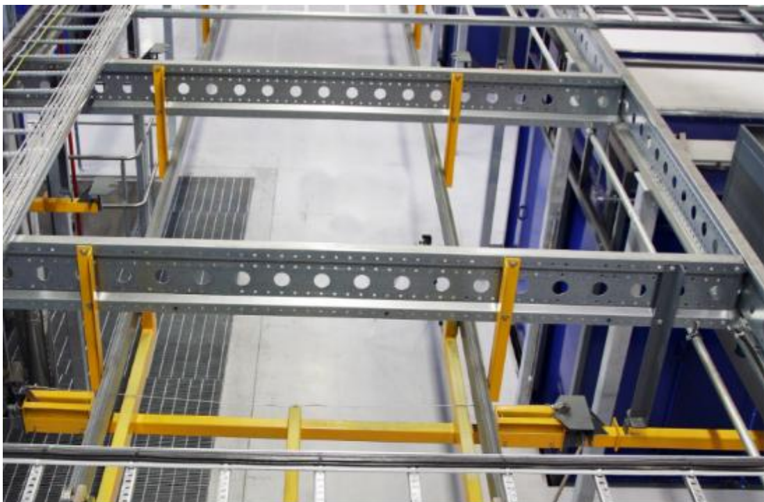
Figure 1-2 CFS channels with web holes used in industry building (Chen et al., 2024)
