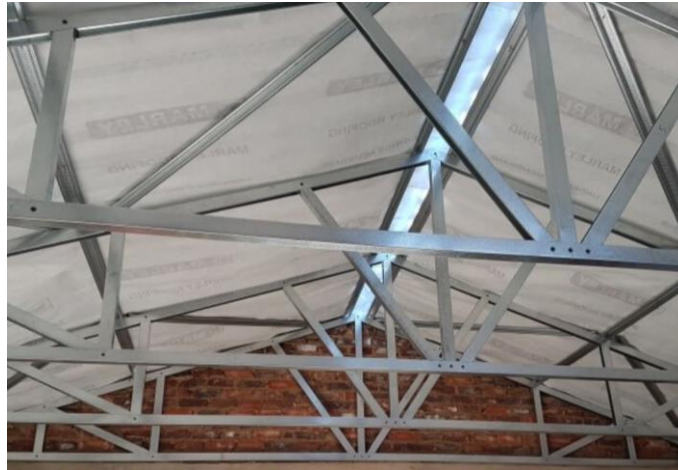
Figure 2-8 HRCs used in roof trusses
