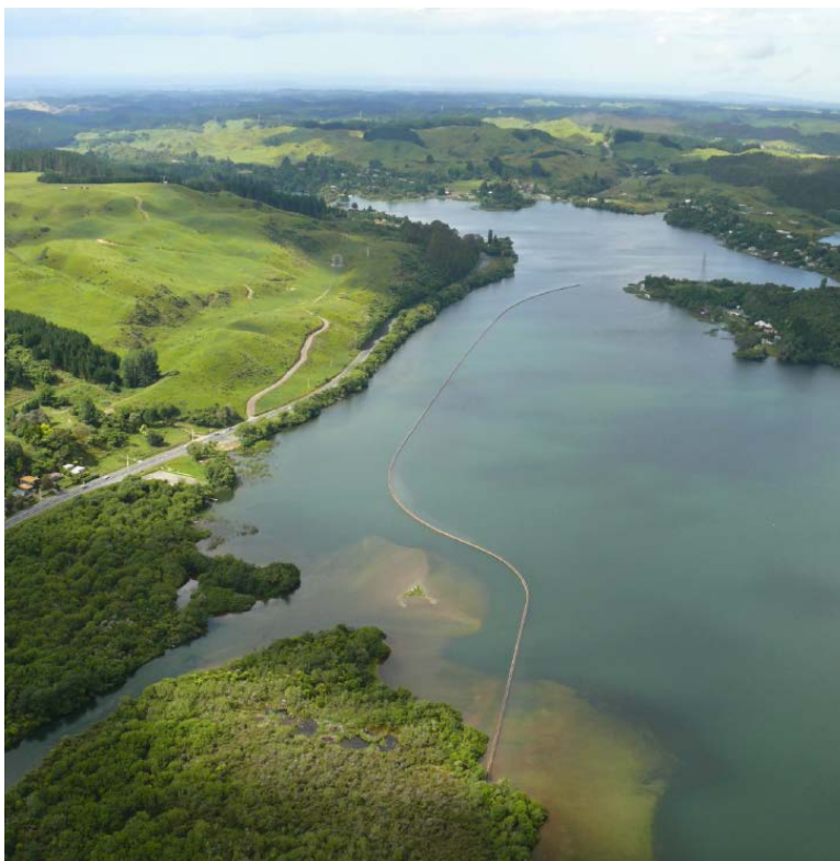
Figure 2-3. Aerial view of the Ohau Channel diversion wall that diverts water from Lake Rotorua towards the Kaituna River outflow (Hamilton et al. 2018).
