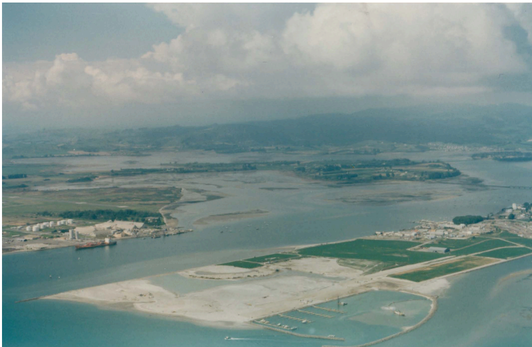
Figure 2.21: Sulphur Point reclamation (looking south-east) during construction of the boat marina in 1981. (Source: Healy, 1985)
