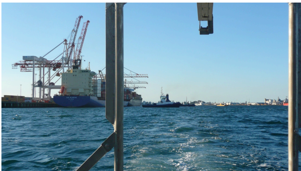
Figures 5.20 & 5.21: Photos of the Port of Tauranga in August 2011 showing the propeller wash from the ship's bow thrusters (top) or the tugboats (bottom). These could explain the deep areas adjacent to the wharves.
