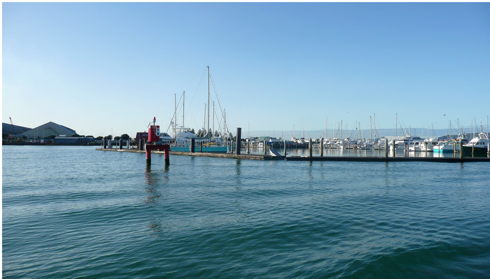
Figure 1.7: Northern floating pontoon of the Tauranga Bridge Marina.
