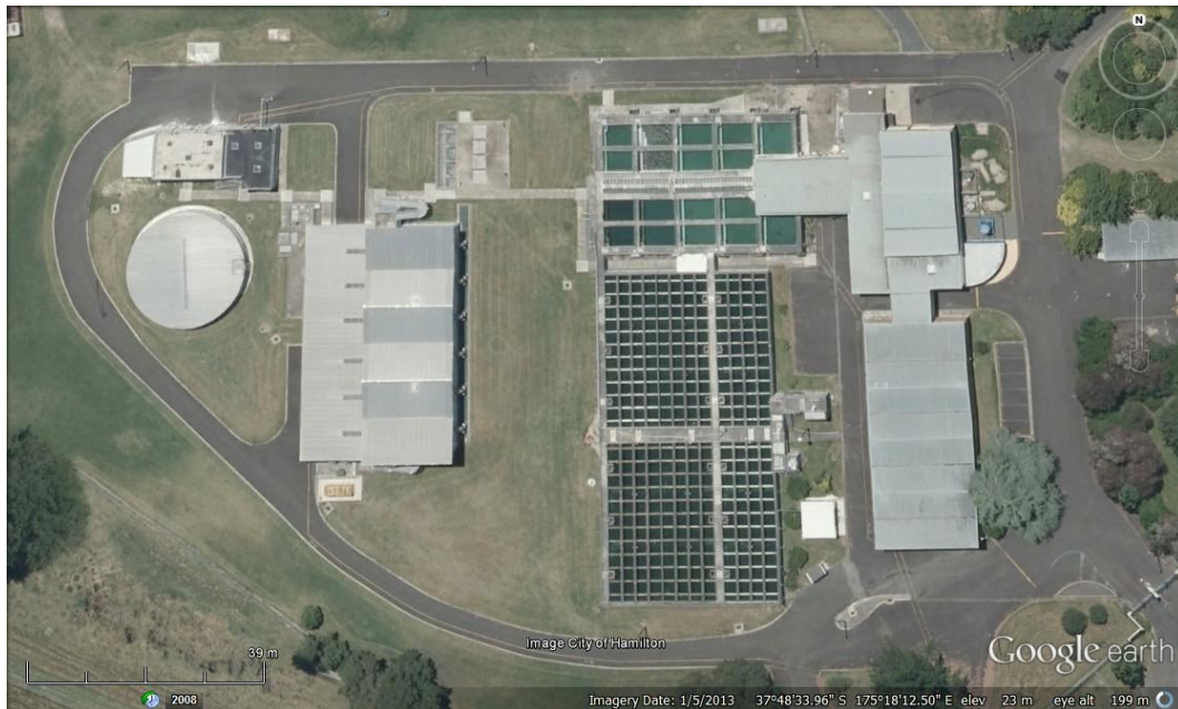
Figure 1-2: Aerial view of the Hamilton Drinking Water Treatment Station (Source: 37°48'33.96" S 175°18'12.50" E. GOOGLE EARTH. January 5, 2013. October 23, 2015).
