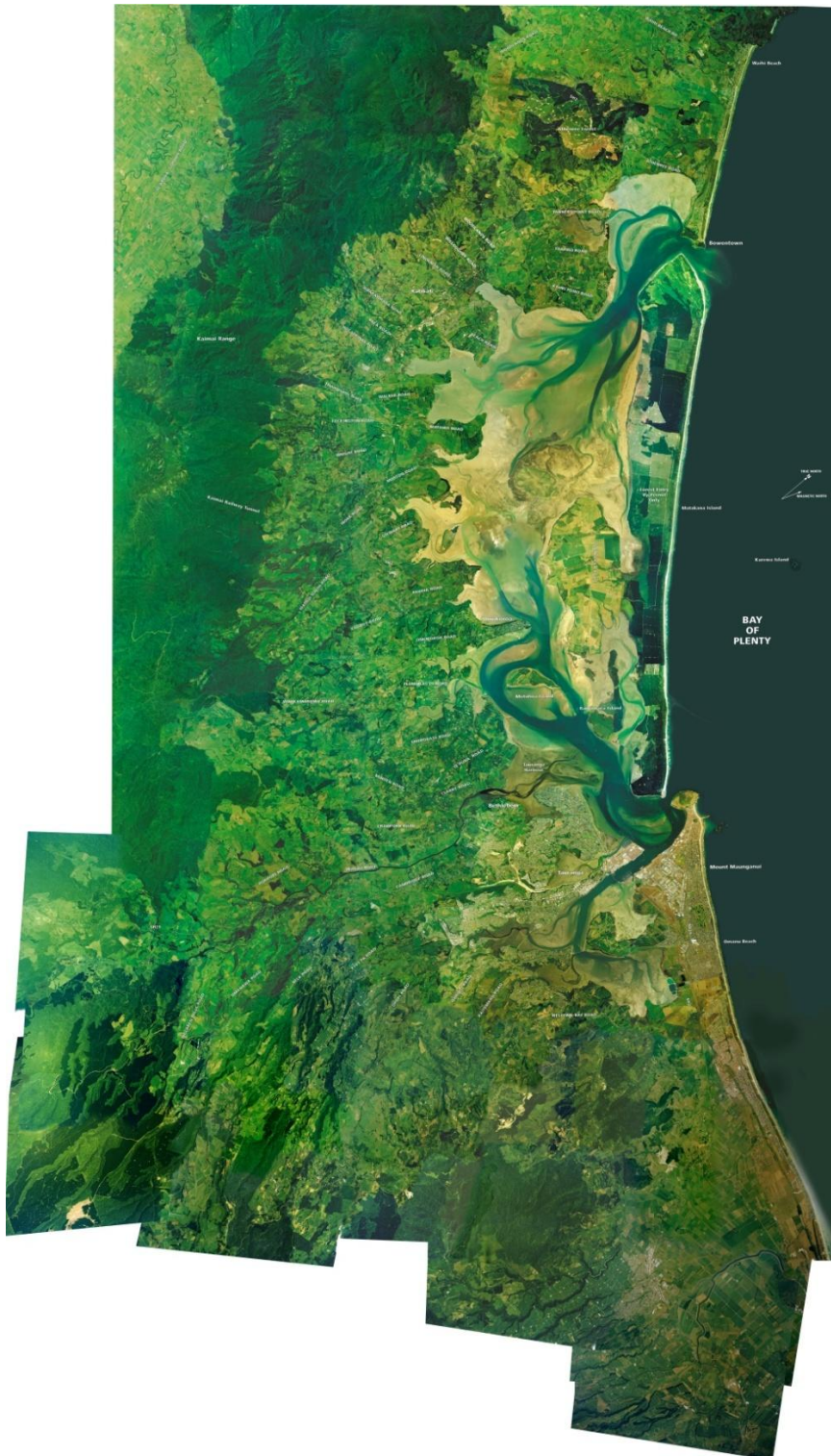
Figure 4.3 Colour Aerial View of the Case Study area, showing the extensive intact indigenous forest of the Kaimai Ranges (upper to mid-left); dendritic gully and riparian vegetation (lower left); and fragmented lowland mixed use landscape (Data produced and supplied by Global Aerial Surveys Ltd, Kaimai 2 Coast).
