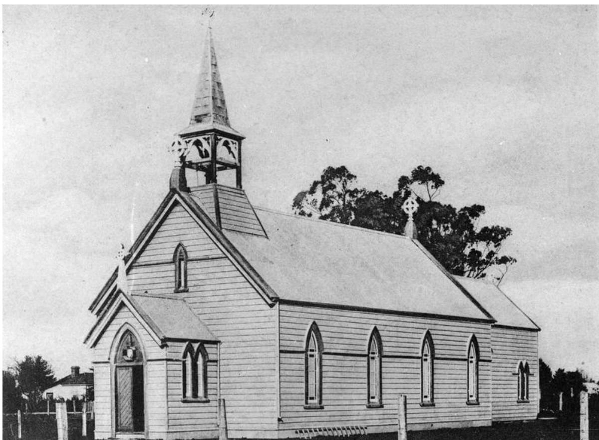
Figure 24 St Mary's Church, Clyde Street, 1890 118
