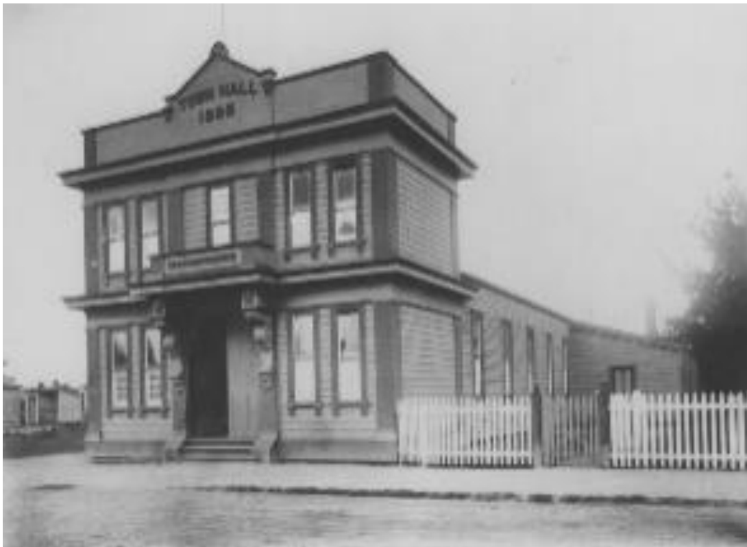
Figure 17 Te Awamutu Town Hall 1895 69
