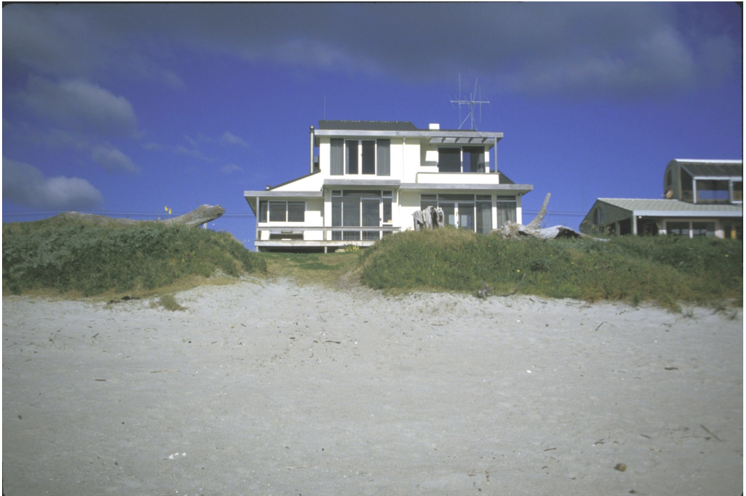
Figure 4. Coastal subdivision much too close to the beach, and deteriorating the amenity and intrinsic value of the beach environment.
