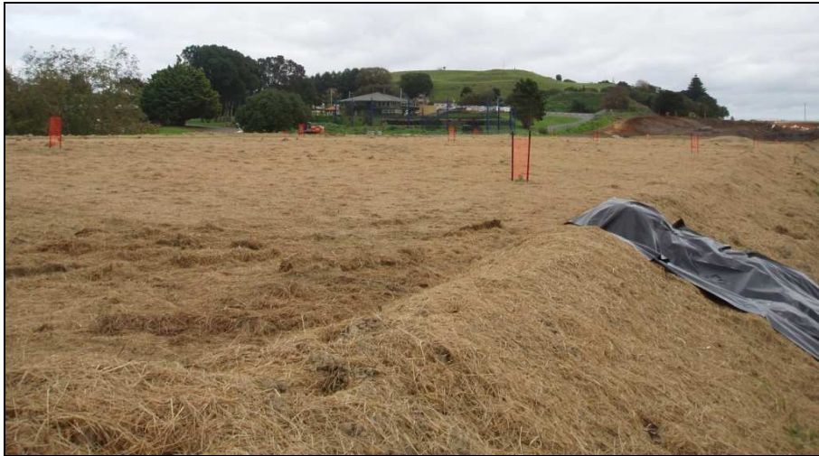
Fig 2.5: Protective hay covering a completed earthworks site.
