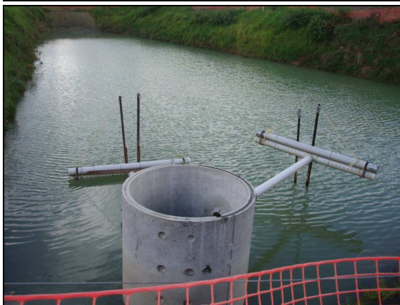
Fig. 5.15c: Following further rainfall and runoff, the water level of the main pond has increased to above the lower decant arm (02/04/07).
