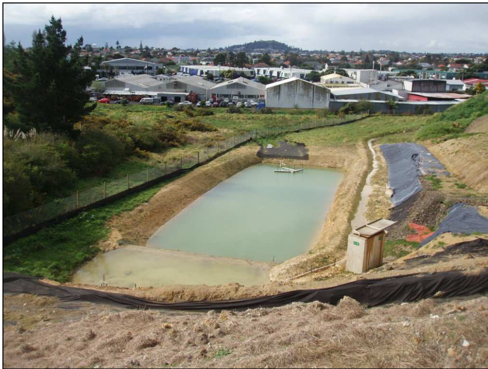
The Richardson Road Sediment Retention Pond in August 2007.
