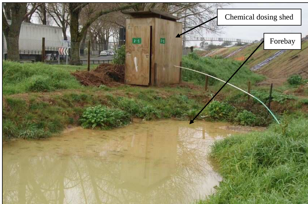
Fig. 2.10: A Chemical Dosing Shed located near the forebay of a sediment retention pond.
