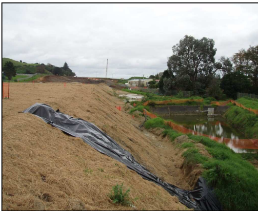
Fig. 3.16a: Mulch applied to all exposed surfaces areas at the Somerset Road pond to reduce erosion.
