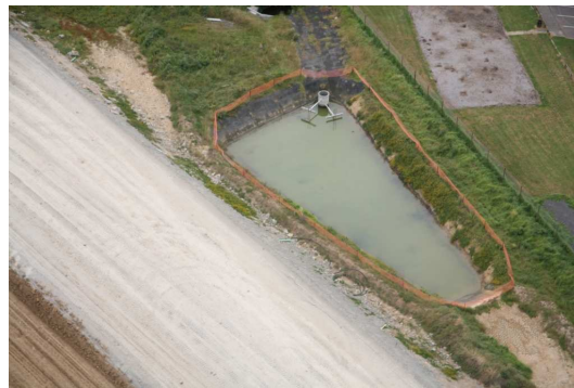
Fig. 6.1b: Aerial view of the onsite works adjacent to the Somerset Road pond in December 2006 (Photo courtesy of Transit, 2006).
