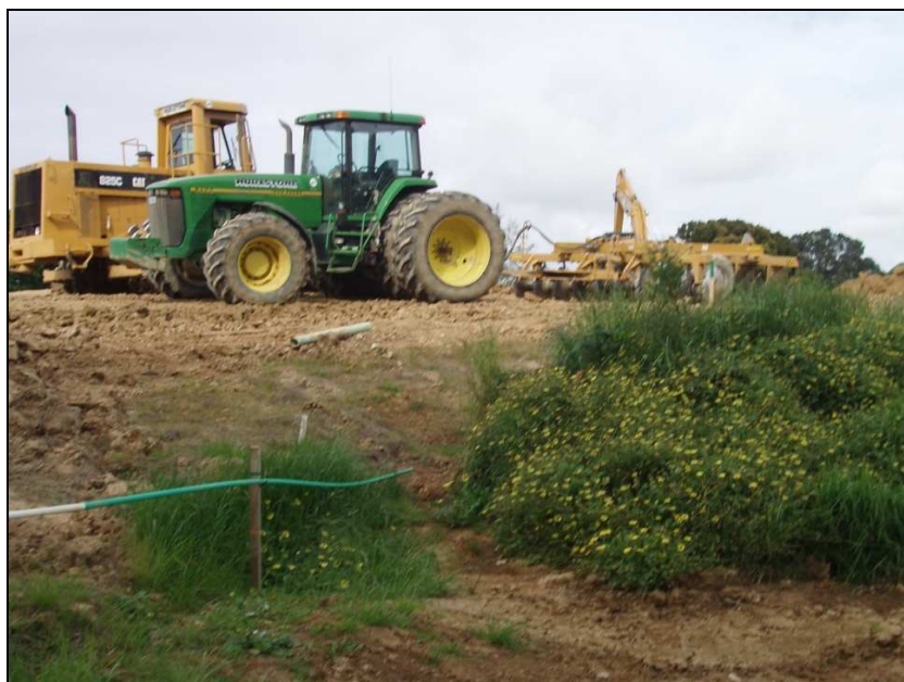
Fig. 2.4: Large earthmoving machinery on an earthworks site.
