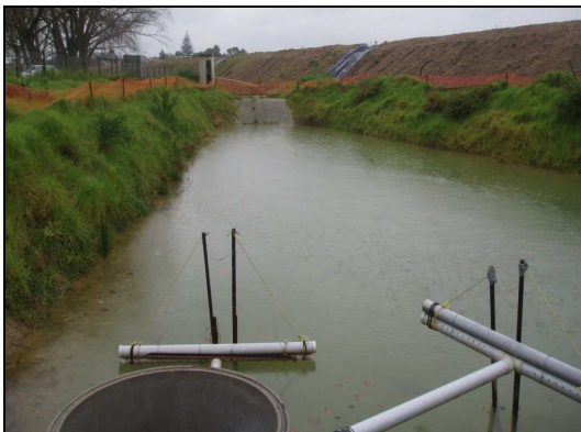
Fig. 3.12a: View of the decanting structure
