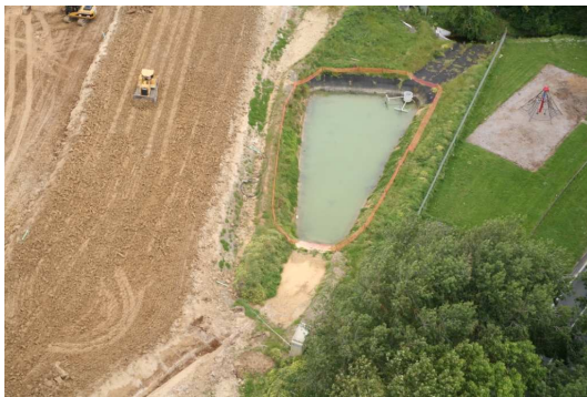
Fig. 6.1a: Aerial view of the onsite works adjacent to the Somerset Road pond in November 2006 (Photo courtesy of Transit, 2006).
