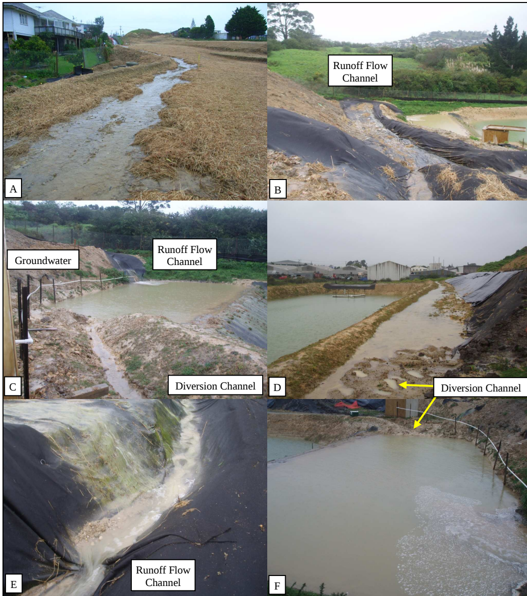
Fig. 6.8: The Richardson Road forebay on 11/07/07 where: A: Preferential flow path across the surface; B: Runoff flow channel to the forebay; C: Location of the forebay diversion and runoff flow channels and the groundwater input; D: View of the diversion channel looking towards the main pond discharge; E: Sediment - laden water flowing down the runoff flow channel; and F: Turbulence in the forebay caused by the runoff flow.
