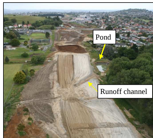
Fig. 5.11b: Earthmoving works in the catchment of the Somerset Road pond on 17/12/06. (Photo courtesy of Transit, 2006).
