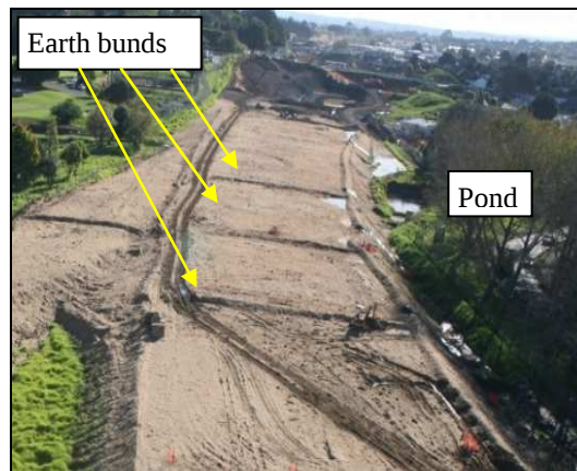
Fig. 3.16b: Earth bunds were used to reduce erosion onsite (Photo courtesy of Transit, 2007).
