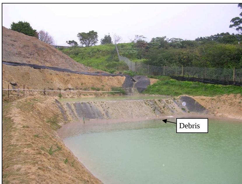
Fig. 5.26: Floating debris at the start of the Richardson Road main pond.
