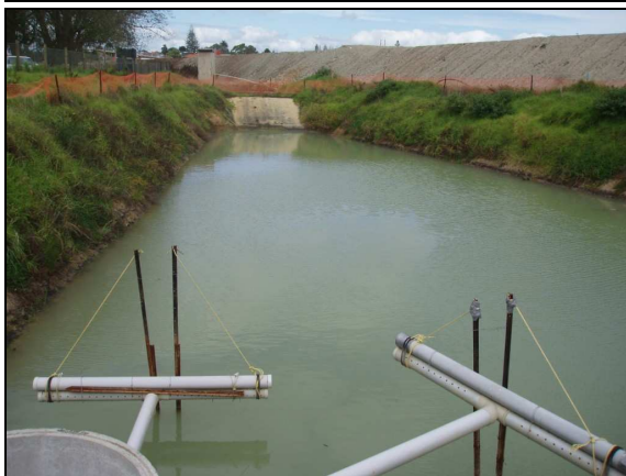
Fig. 5.15b: Heavy rainfall has resulted in runoff, and thus an increase in water levels in the main pond (21/03/07), reducing the gap between the water level and decant.
