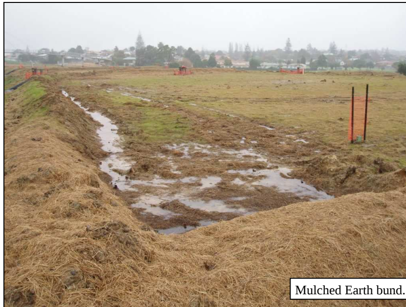
Fig. 6.2: Earth bunds and mulch were used to slow the flow of runoff and aid the establishment of grass. Water has ponded against the earth bund rather than flowing down the bank.
