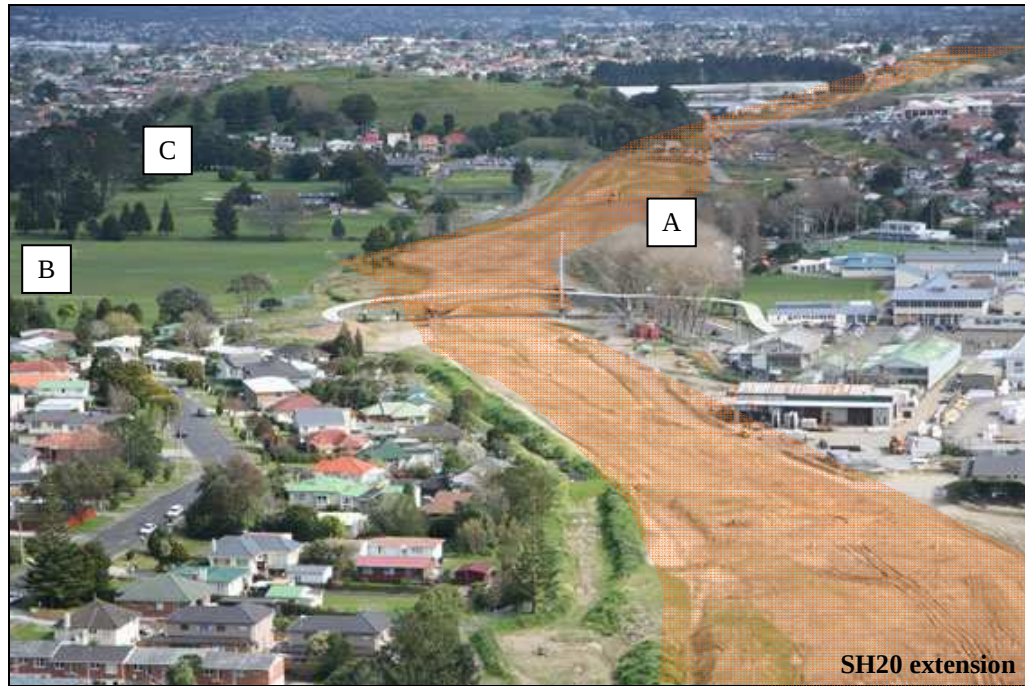
Fig. 3.8: Aerial view of part of the SH20 extension showing; A: the Somerset Road pond, B: Keith Hay Park, and C: Akarana Golf Course (Photo courtesy of Transit, 2007).
