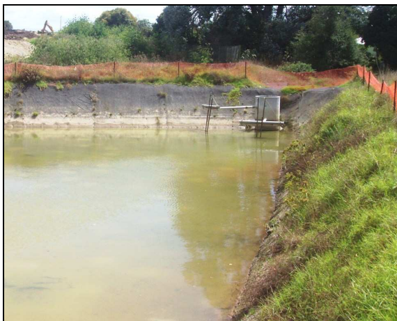
Fig. 5.15a: Very low water level in the main pond (05/03/07). The gap between the decant and water level is approximately 30cm.
