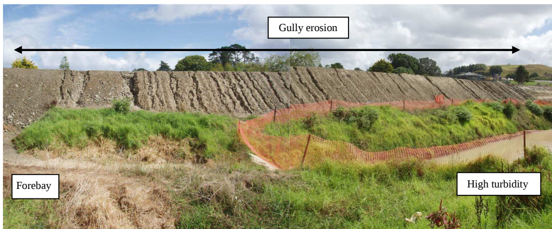
Fig. 6.5: Pronounced gully development in the banks alongside the Somerset Road pond, and high turbidity levels are apparent in the main pond.
