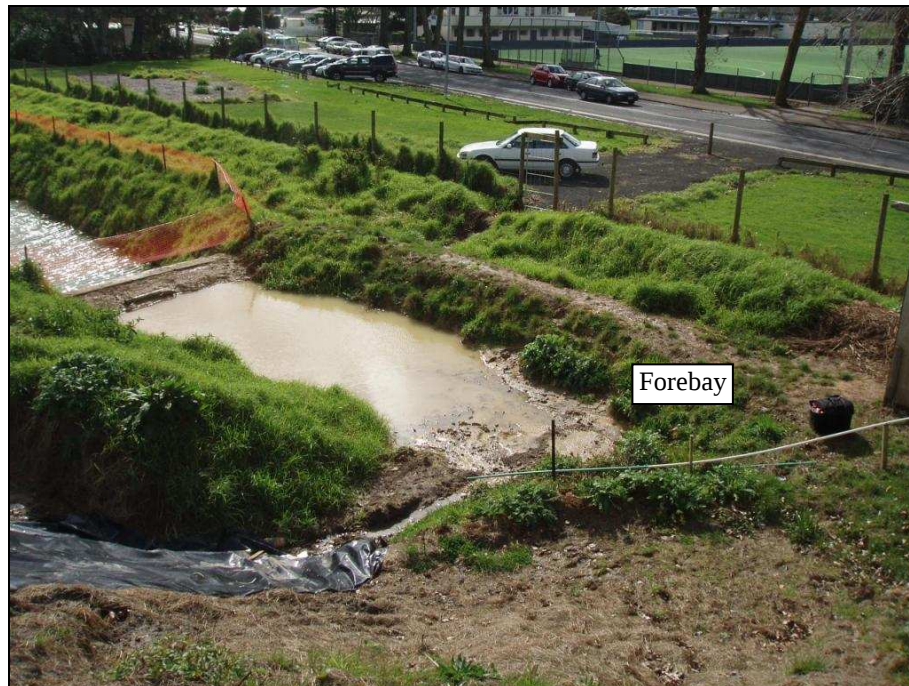
Fig. 5.13: View of inlet to forebay showing high levels of suspended sediment in the water.
