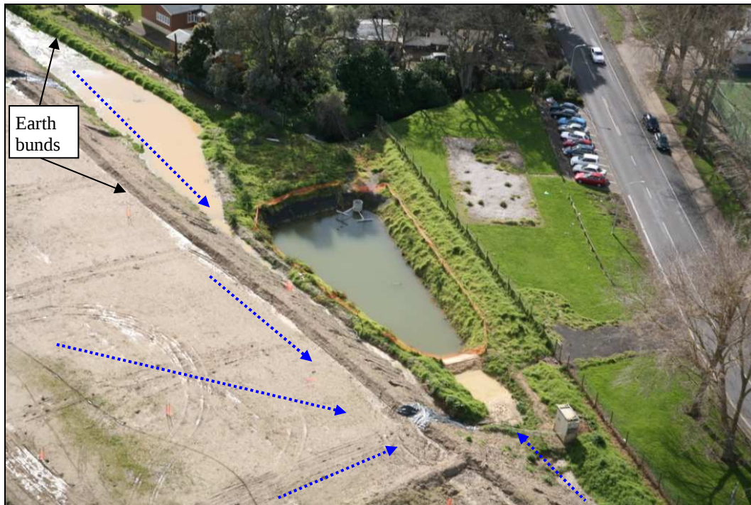
Fig. 3.13: General flow direction towards the Somerset Road pond (Photo courtesy of Transit, 2007).
