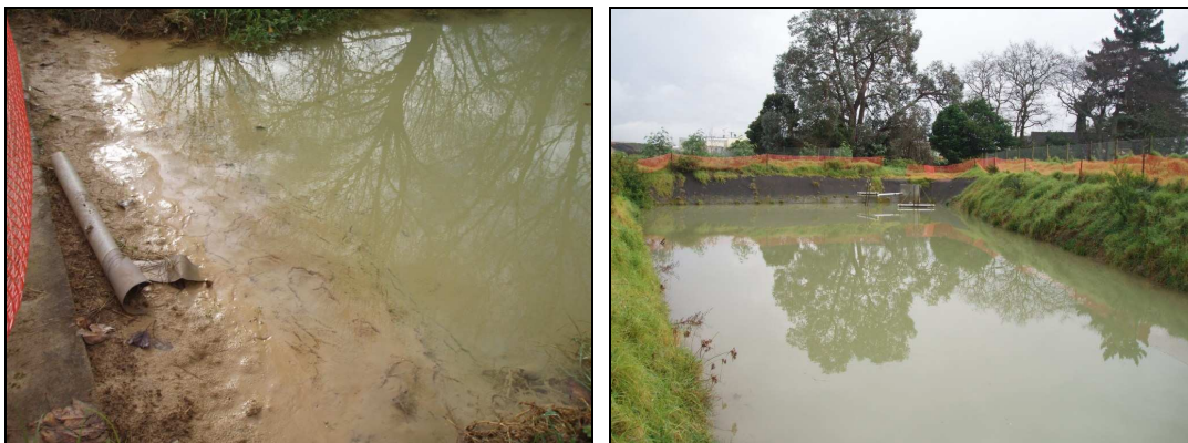
Fig. 5.17a: Clear water in the forebay (01/08/07). Fig. 5.17b: Turbid water in the main pond (01/08/07).
