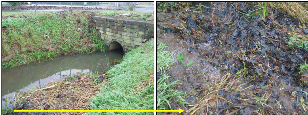
Fig. 5.39: View of the Downstream B site, showing the culvert beneath Somerset Road, and the sludgy sediment beside the stream (inset).
