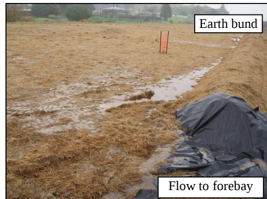
Fig. 5.9b: Earth bund and mulch. Note the stabilised entrance to the forebay.
