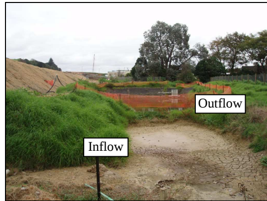
Fig. 5.8b: Damp mud in the Somerset Road forebay on 16/05/07 following earlier rainfall.
