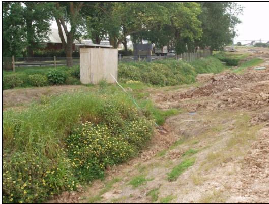
Fig. 3.11a: Unstabilised entrance to the Somerset Road pond, November 2006.
