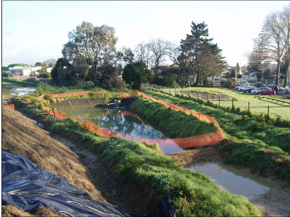
The Somerset Road Sediment Retention Pond on a crisp July morning 2007.
