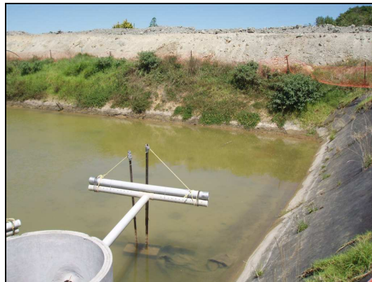
Fig. 5.14b: Water quality in the Somerset Rd pond on 26/02/07. Note the low water level.
