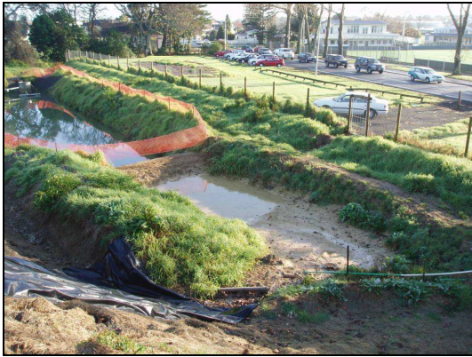
Fig. 6.4a: Water accumulated in the lower “outflow” portion of the Somerset Road forebay on 26/07/07.
