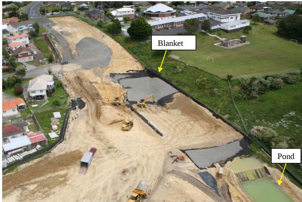
Fig. 3.23: Aerial image of the installation of the drainage blanket (black) upslope of the Richardson Road pond. The aggregate is currently being added (grey) (Photo courtesy of Transit, 2006).
