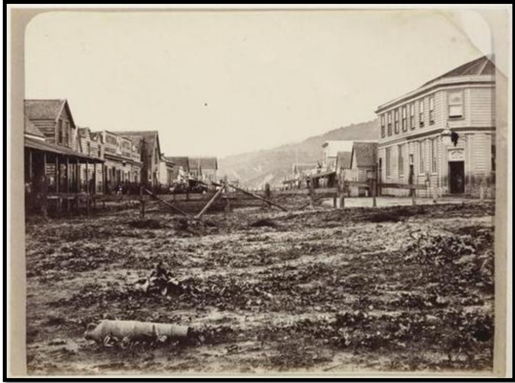
Figure 3: View of Pollen Street dated early 1870s, illustrating the poor state of the town's roads. 175
