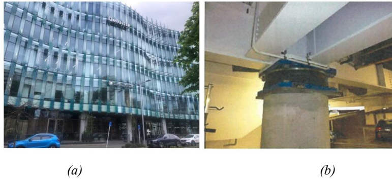
Figure 6. 151 Cambridge Terrace: (a) Global view (Courtesy of Lianyan Li), (b) Base-isolator (Courtesy of Mark Willard).
