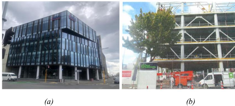
Figure 7. Awly Building: (a) Global view (Courtesy of Lianyan Li), (b) Hybrid structure during construction in March 2016 (Courtesy of Mark Willard).
