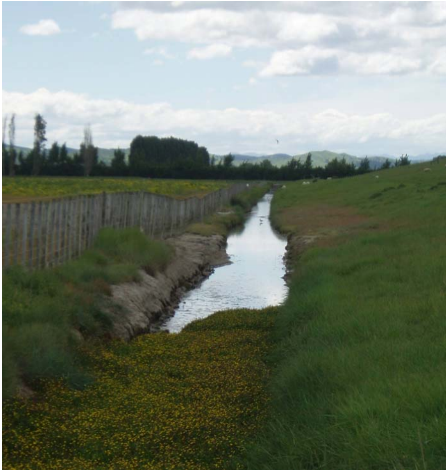
Figure 3.15: Perimeter Drain adjacent to the Gavin's Block.
