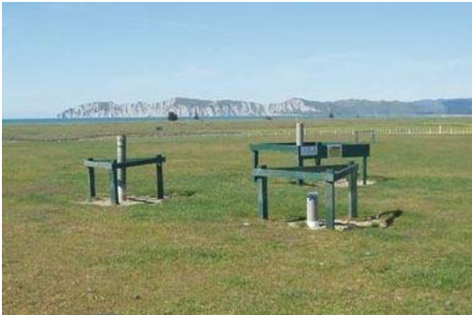
Figure 4.2: Leachate bore 2 and groundwater bores 404A and 404B.
