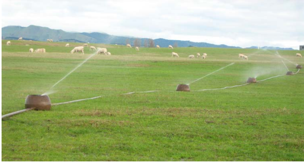
Figure 3.11: Leachate sprinkler line showing “K line” sprinklers.
