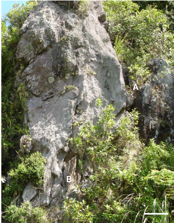
Figure 4.6 – Indurated andesite outcrop exhibiting wide discontinuity spacing. The relaxed state of the discontinuities produces some extremely wide apertures as seen in the upper right of the figure where shrubbery is growing within the discontinuity (indicated by ‘A’). Note the slaty habit of the indurated andesite displayed nearer the base of the outcrop (indicated by ‘B’). Photo taken at site 29. White bar represents 1 m.
