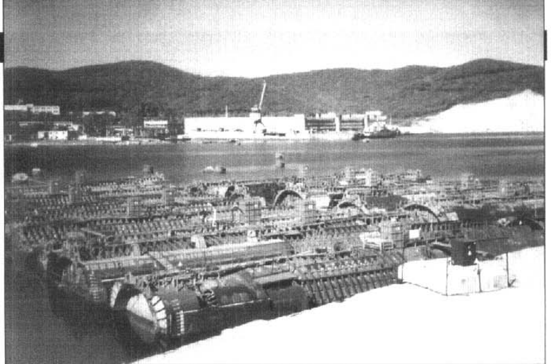
A platform for the temporary storage of submarine reactor compartments in Primorski Krai
