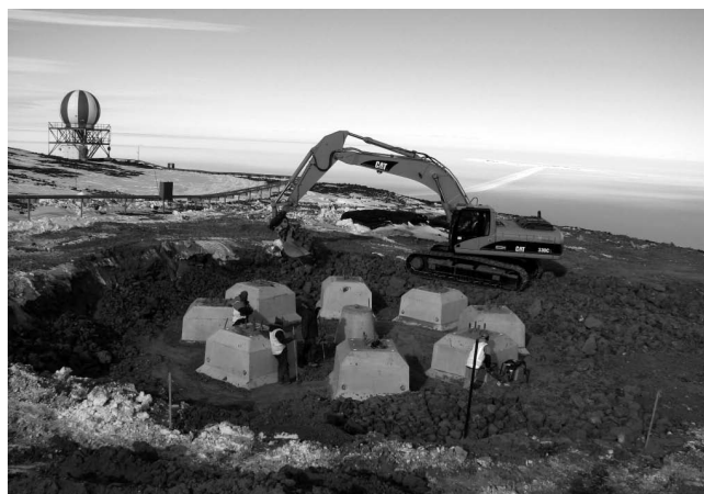
Foundations going in for the proposed windfarm site on Ross Island, Antarctica. (Photograph provided by Megan Balks)
