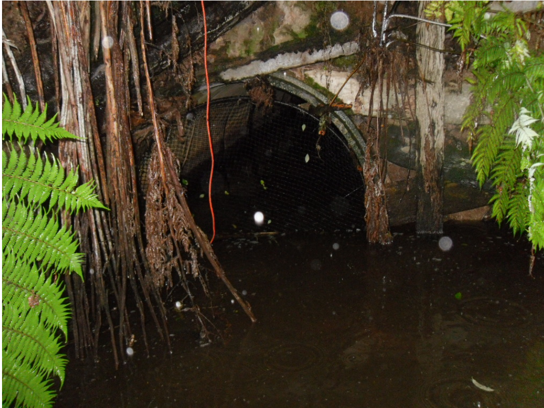
Figure 6. Temporary adult fish barrier installed on the Lake Ohinewai drain on south side of the Tahuna Road culvert 15 January 2011. Photo: A. Daniel.
