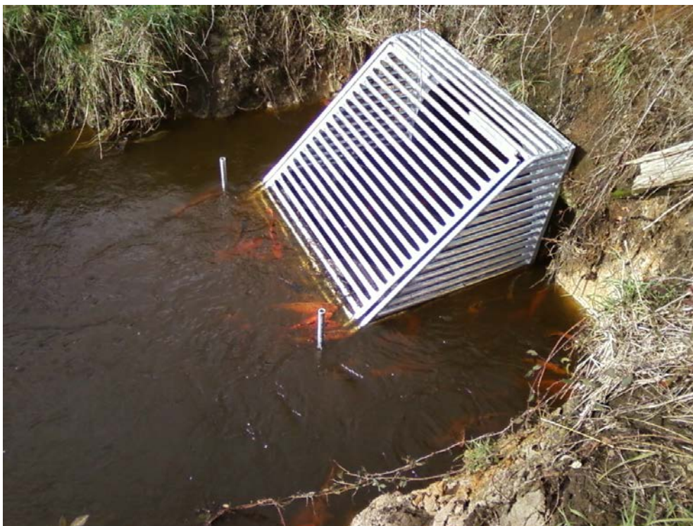
Figure 13. Approximately 60 koi carp attempting to enter to pass the adult pest fish barrier on the Lake Ohinewai Drain. Photo: A. Daniel.
