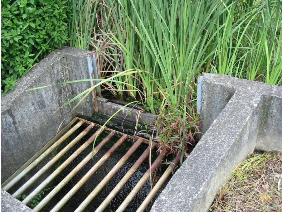
Figure 7. Structure at the downstream outlet of Lake Rotokaeo, Hamilton, that is most probably a barrier to upstream migration of fish species other than eels.
