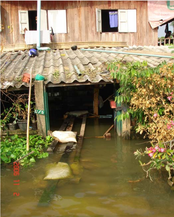
Figure 19 Local eating place submerged under water
