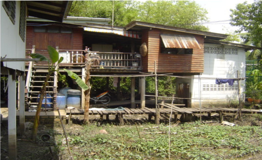
Figure 16 Two level homes on posts
