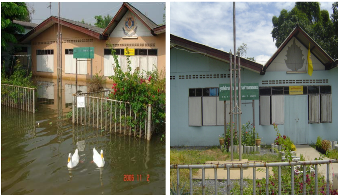
Figure 18 Flooded Early Childhood Development Centre (November 2006), and after clean up and rehabilitation (May 2007)
