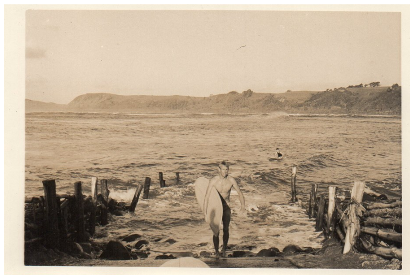
Figure 7.4: Early boat ramp at Manu Bay (Image courtesy of Puriri (2015 b)).
