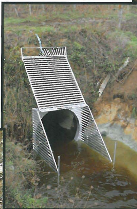
Figure 1. Pest fish exclusion barrier installed on the Lake Ohinewai outlet. The barrier is designed to allow one-way passage of pest fish species out of the lake. Photos: Adam Daniel
