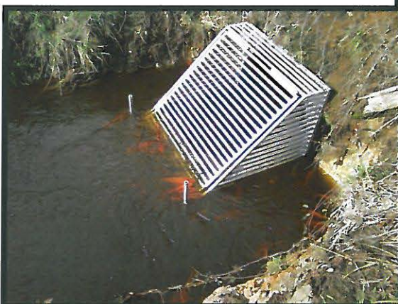
Figure 1. Pest fish exclusion barrier installed on the Lake Ohinewai outlet. The barrier is designed to allow one-way passage of pest fish species out of the lake. Photos: Adam Daniel
