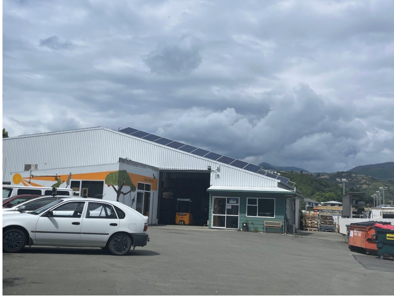
Figure 3.1: Chia Sisters Factory in Nelson with a solar array on the roof.
