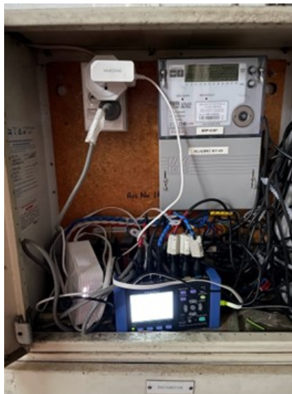
Figure 3.6: A view of the completed setup installed at Chia. This figure shows the data logger and the Linux box installed at Chia Sisters.
