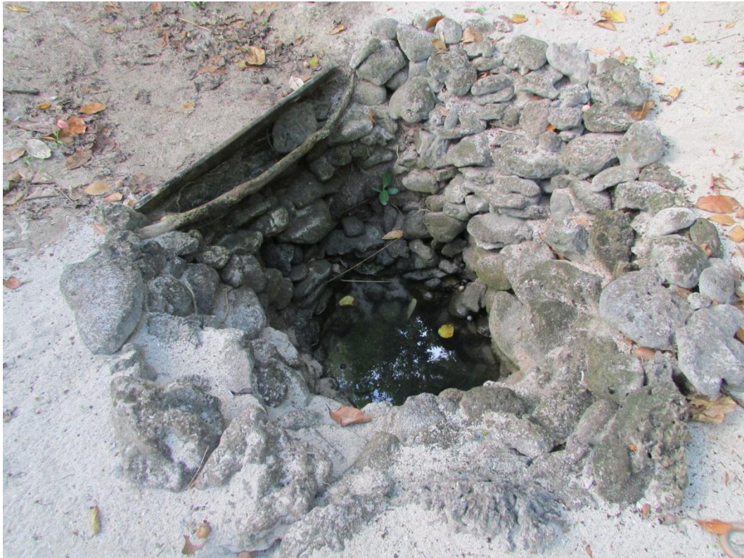
Figure 9: Water source for the Naro community which is vulnerable to saltwater intrusion and drying up during dry season. Photo source: author.
