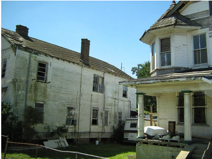
Photo 2- Photo depicting the heavy damage to houses caused by aftermath Katrina in the Lower 9 th Ward, New Orleans (Photo by Jo Barnes).
