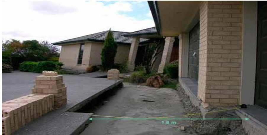
Photo 5: A house in Kaiapoi moved on its foundation in both the September and February earthquakes a total of 1.8m (photo: Lai). Source (EERI, 2011).
