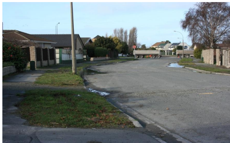
Photo 4: An abandoned street beside Avon River in Christchurch 2012. Seen in the background is a truck driving towards a construction site to load up demolition debris. (Photo taken: 03/8/2012 by Sue Chaytor).
