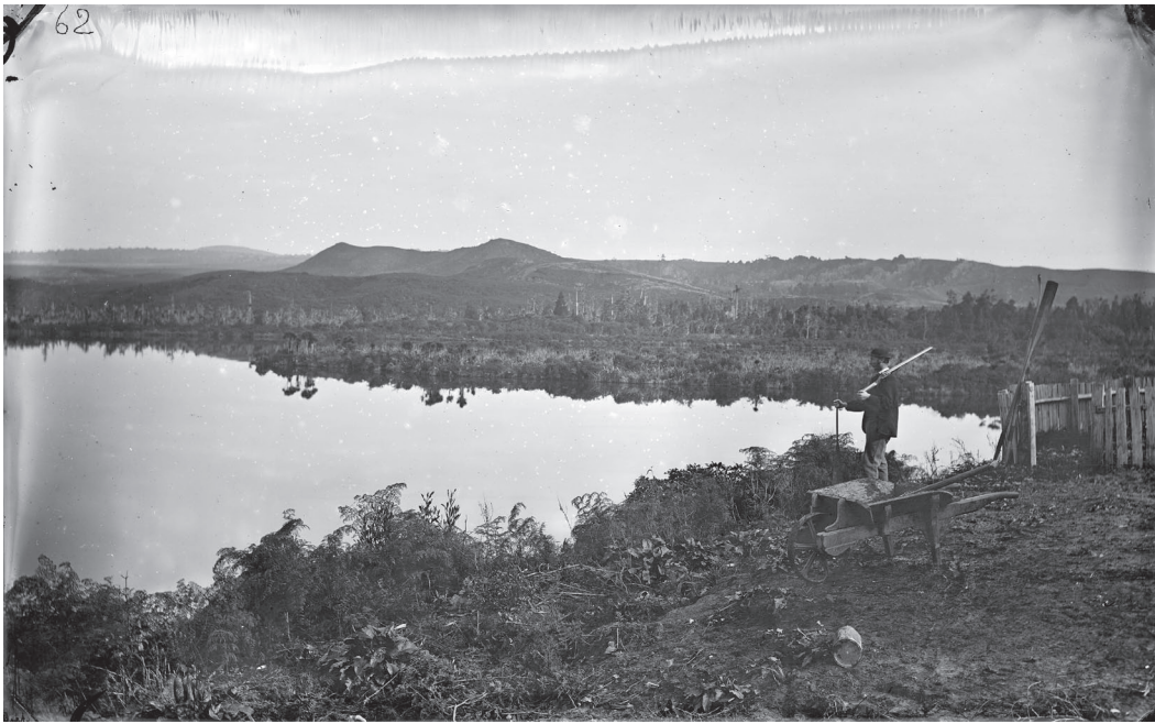
Fig 5.4 Scene near Whangamarino bridge
