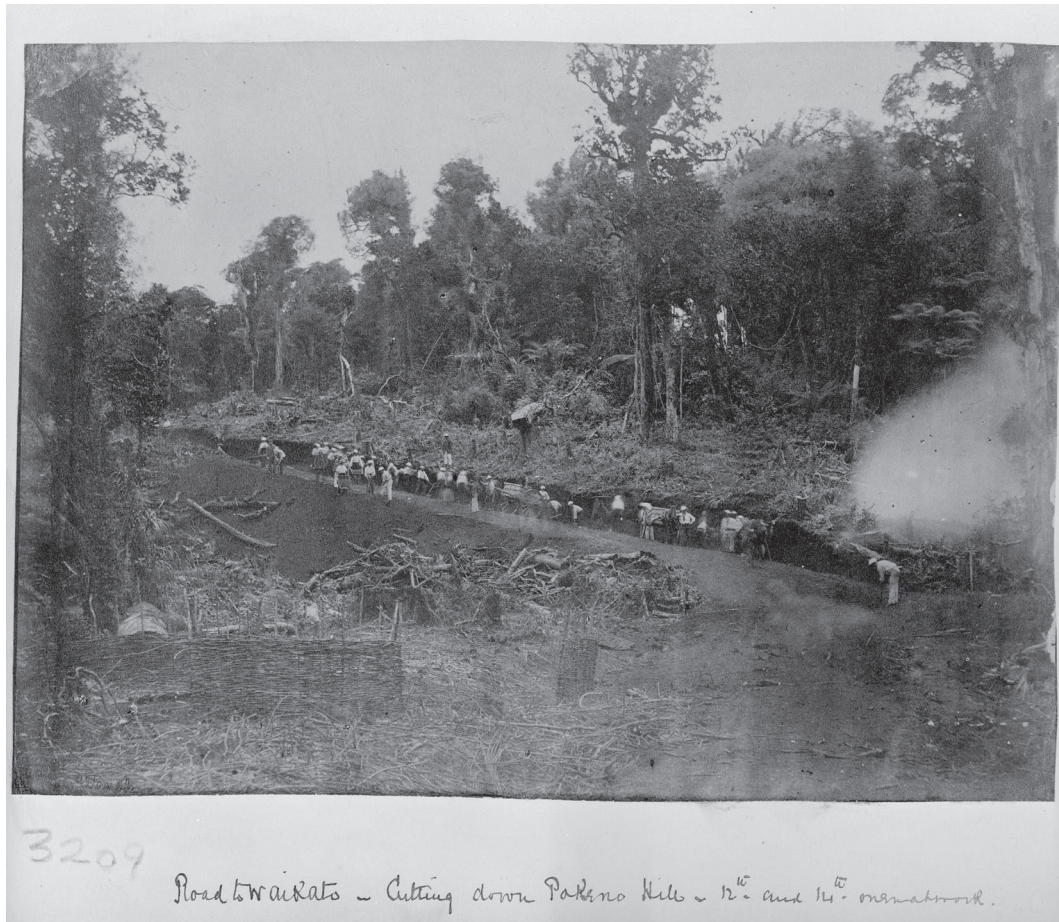
Fig 4.3 Construction of a road to Waikato, Pokeno Hill
