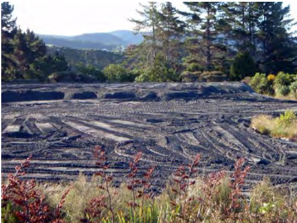
Figure 10.11. In-filling the saltmarsh using marina dredgings
