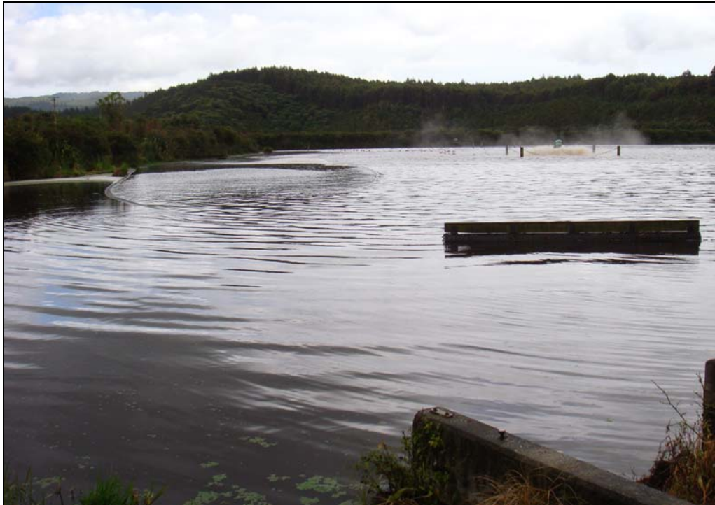
Plate 3.1. Final treatment pond at the Tasman site.
