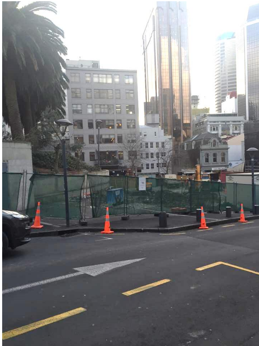
Figure 10. Construction on High Street, Auckland.
