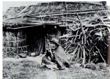
FIG 2: This nineteenth century whare, made of loosely bound reeds with a sack cloth for a doorway, reflects the pragmatic old-time Māori also dressed in the same cloth. The kuia Mata Kukae, pictured here with her smoking pipe, was over 100 when this was taken and died within months (King 1992:92).
