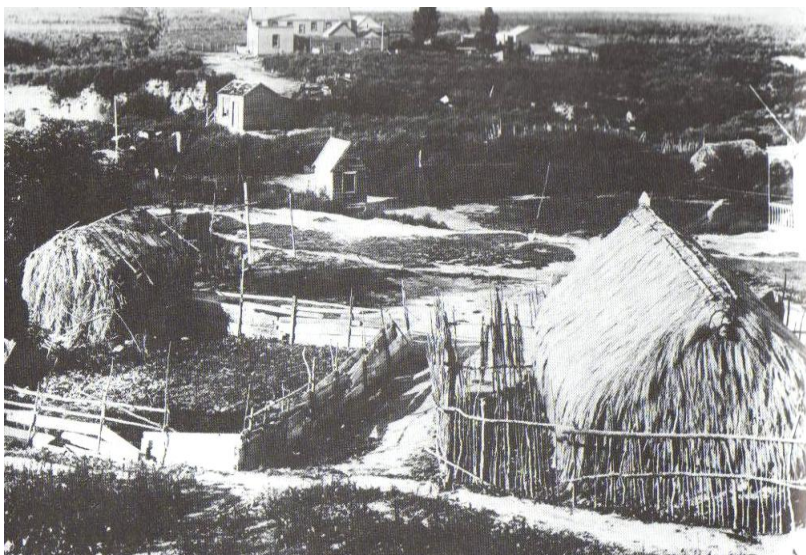
FIG 15: In this late nineteenth century photo of Whakarewarewa at Rotorua, King states "A juxtaposition of traditional Māori and conventional European housing..." Although the whare are no longer as squat as in previous times, they were still made of thatching with earth floors and particularly rudimentary in contrast to the modern housing also evident (King 1996:90)
