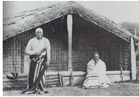
FIG 8: An 1885 Burton Photograph that reflected the proficiency of Kingitanga Māori. Here is a excellent made, securely bound, raupo whare with flax roof. According to King, the standing is the Kawhia Chief Whitiara (King 1992:92).
