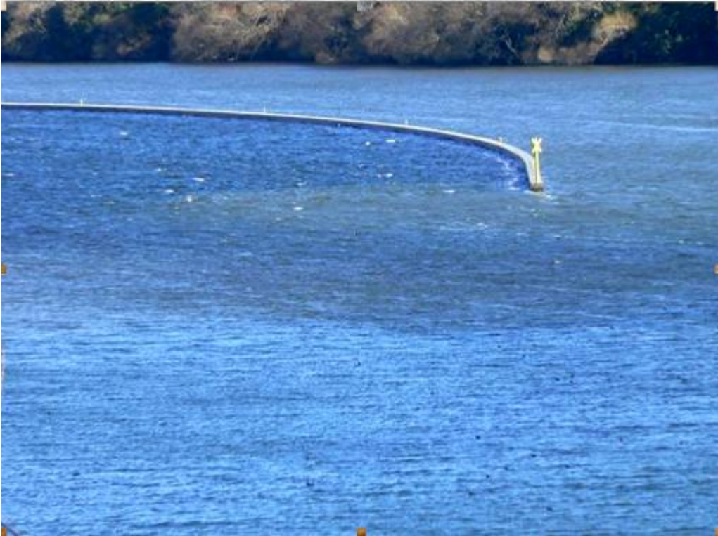
Figure 8. Photo of the end of Ohau Channel Diversion wall taken 13:40 hr on 24 July 2008. Note relatively turbid water from the diversion channel (left-hand side of photo) flowing into relatively clear water of Lake Rotoiti. Photo courtesy of N. Miller.
